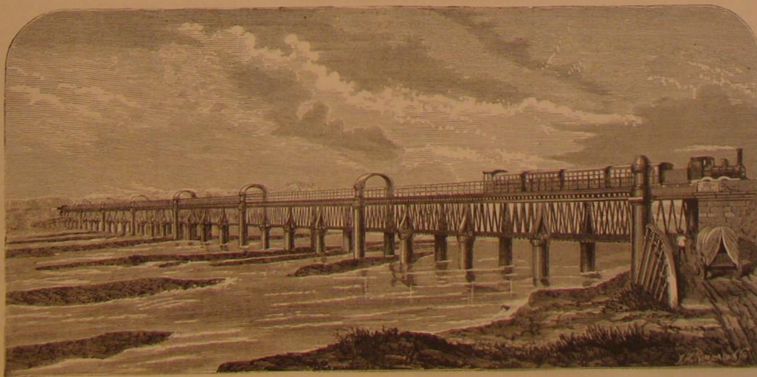
BRIDGE OVER THE WAITAKI NEW ZEALAND.
