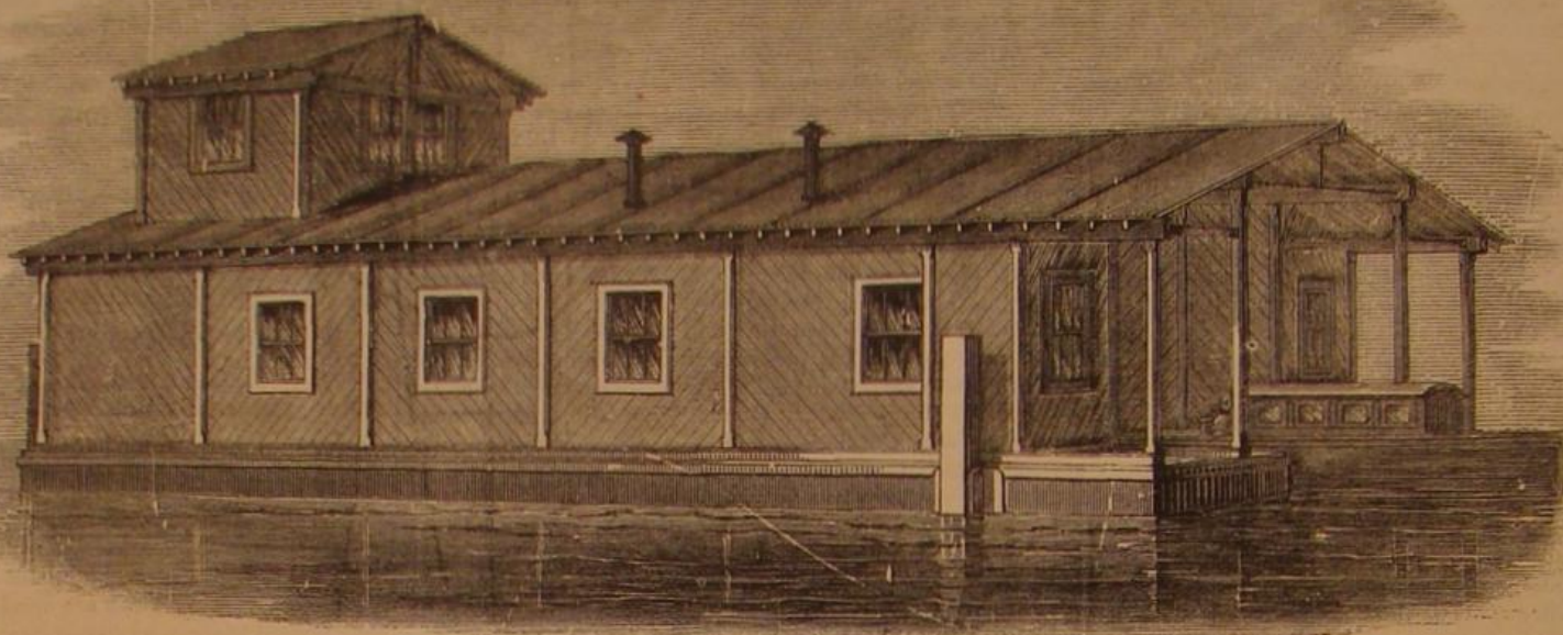
FLOATING STATION FOR FLOATING FIRE ENGINES.
