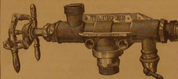
FIG. 1.—THE CLIPPER INJECTOR.
