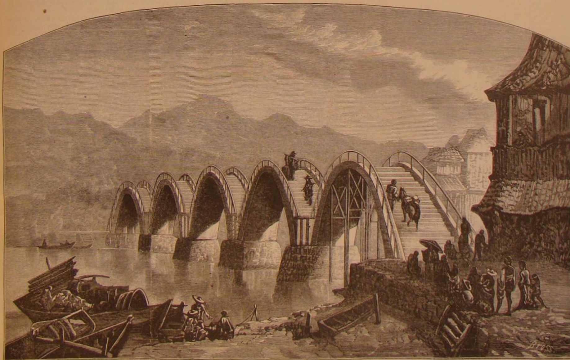
A CURIOUS BRIDGE AT IWAKUNI JAPAN.
