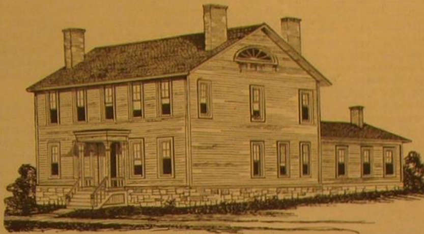
VIEW BEFORE ALTERATION.
