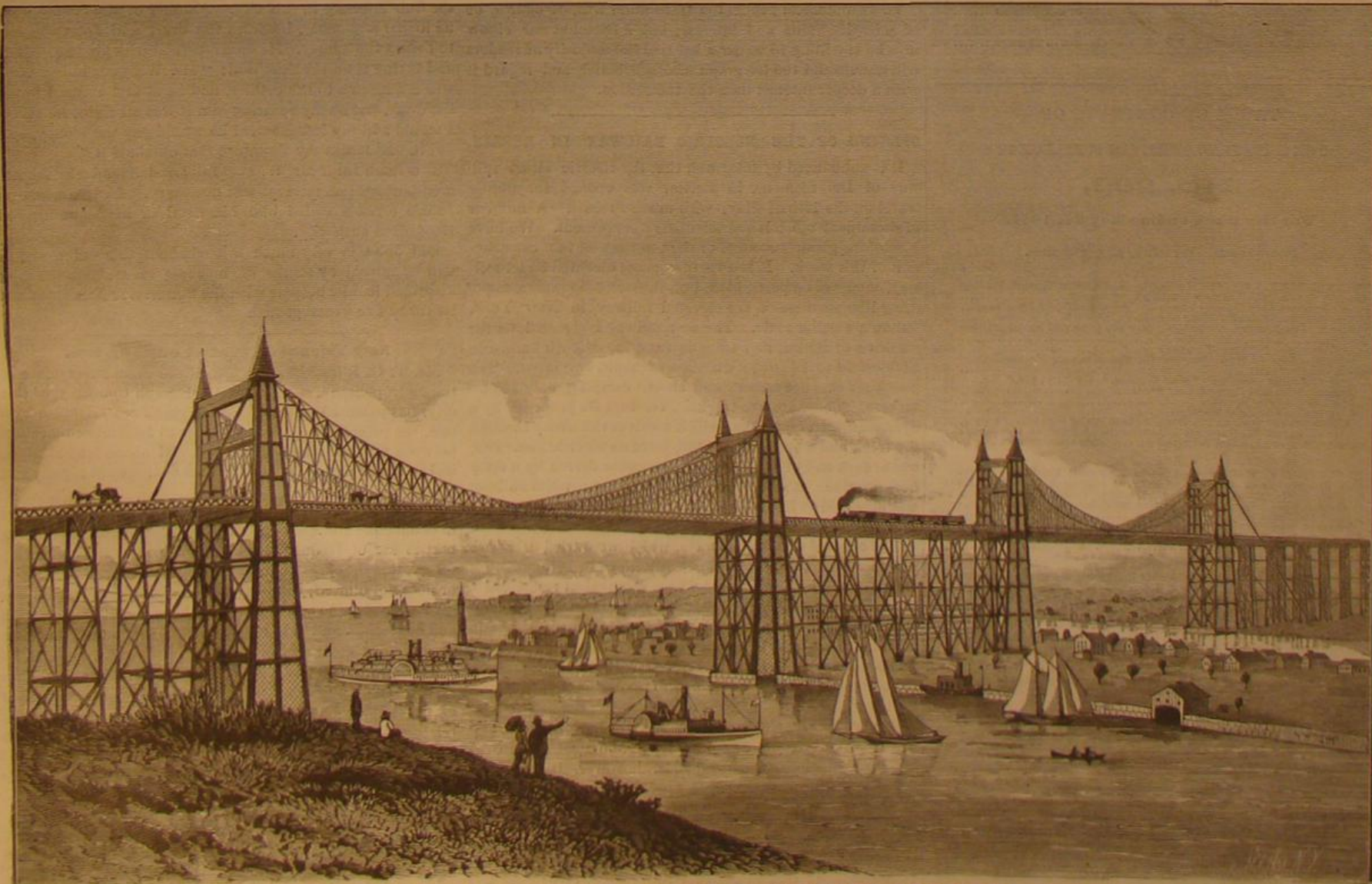
THE SECOND BRIDGE BETWEEN NEW YORK AND BROOKLYN.—OVER THE EAST RIVER AT BLACKWELL'S ISLAND.
