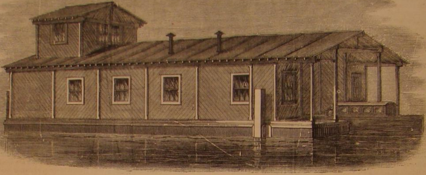
FLOATING STATION FOR FLOATING FIRE ENGINES.
