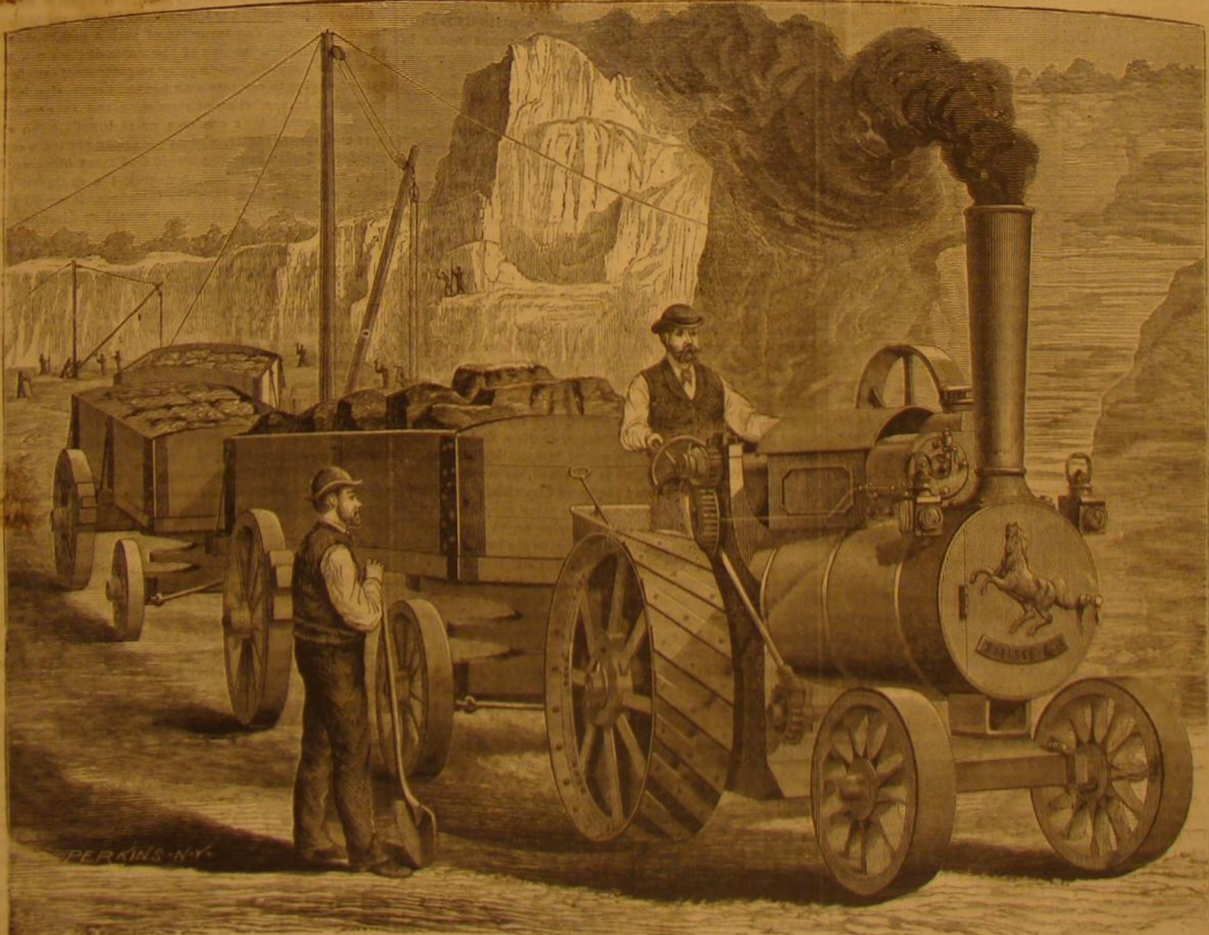
AVELING & PORTER'S ROAD AND FARM LOCOMOTIVE AND WAGONS.
