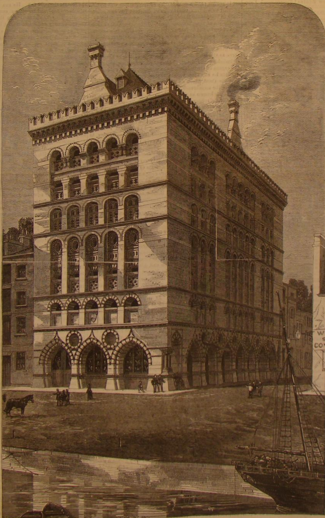
NEW GRANARY AT BRISTOL ENGLAND.
