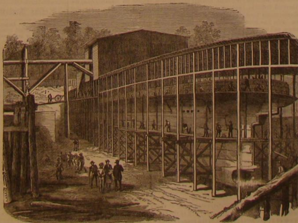
THE STEVENS BATTERY IN THE DRY DOCK, HOBOKEN, N. J.
