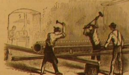
FIG. 12.—RIVETING A COLUMN.
