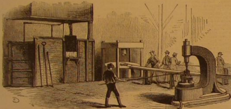
FIG. 13.—FURNACE AND HYDRAULIC DIE.
