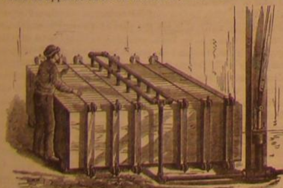
Fig. 4.—PRESSING THE WATER FROM THE SLIP.
