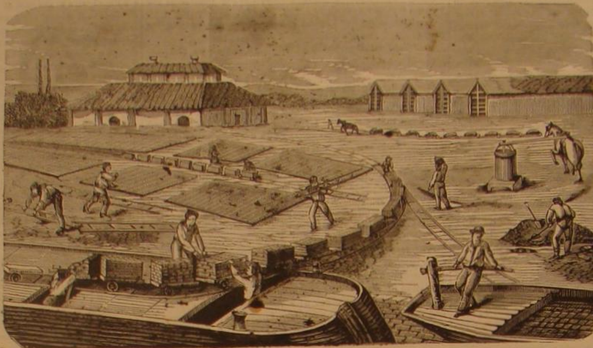
PORTABLE RAILWAY IN A BRICKYARD.
