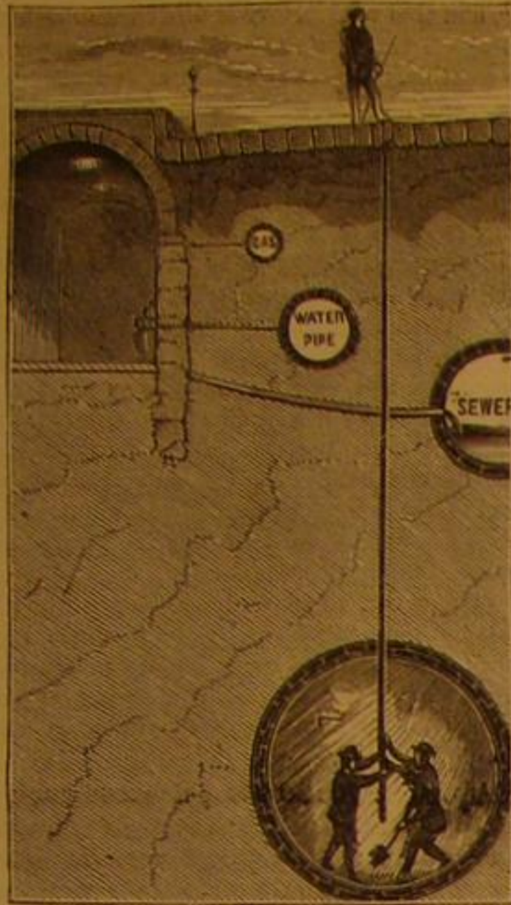
THE TUNNEL AND WAITING STATION.
